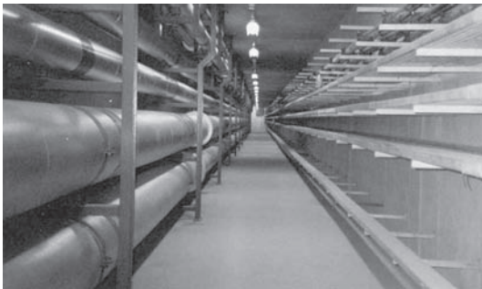
Figure 12.20 Services tunnel
