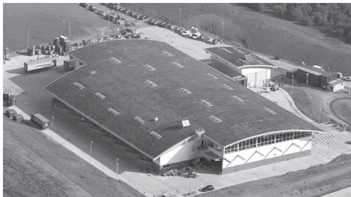
Figure 3.7 Low energy storage building: Adnams Brewery Distribution Centre, Suffolk, UK
