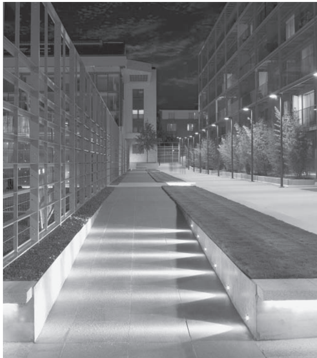
Figure 9.6 Example of a successfully lit and energy efficient external space: Highbury Square, London
