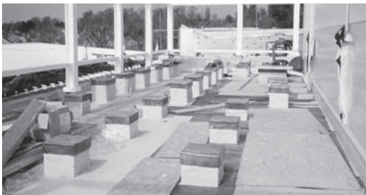
Figure 12.24 Builder's work bases for large air-handling units
